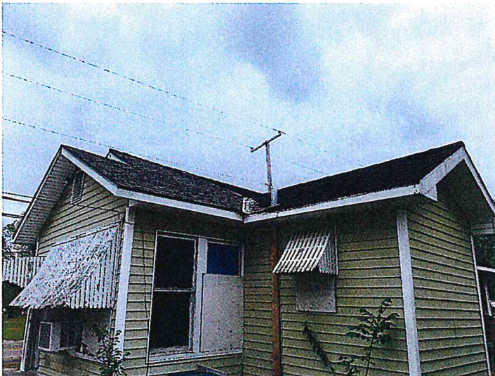
4/19/2016 SAMPLES S55 & S56 - SHINGLE ROOF & FELT MTRL Pic (57).jpg
