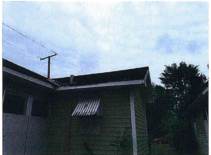
4/19/2016 SAMPLES S47 & S48 - TRANSITE ROOF SHINGLES Pic (58).jpg
