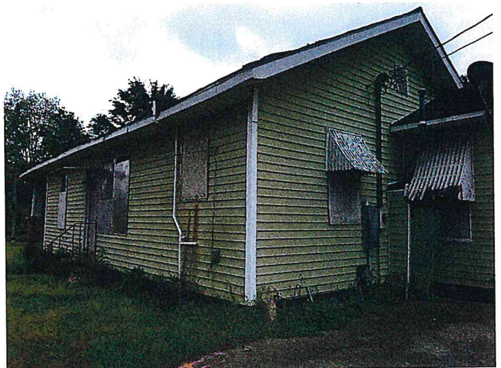
4/19/2016 EXTERIOR SIDE D - 521 A&B NE EVANGELINE THRUWAY Pic (42).jpg
