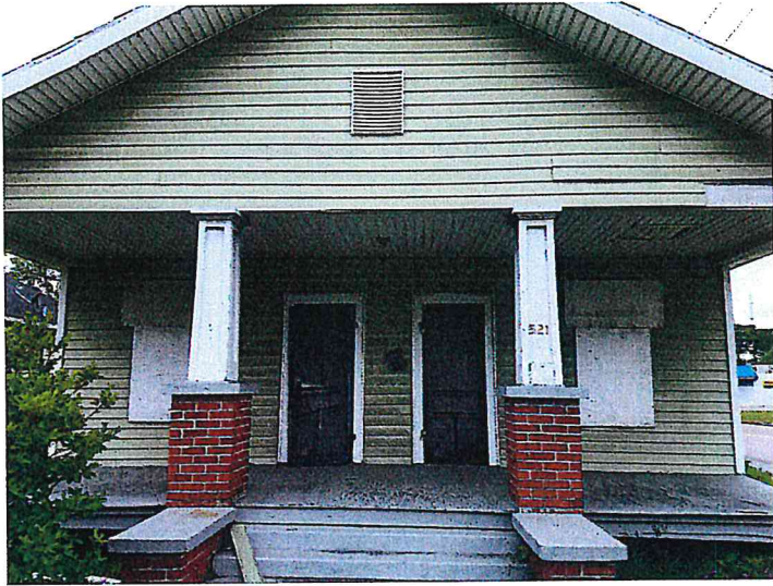
4/19/2016 EXTERIOR SIDE A - 521 A&B NE EVANGELINE THRUWAY Pic (39).jpg
